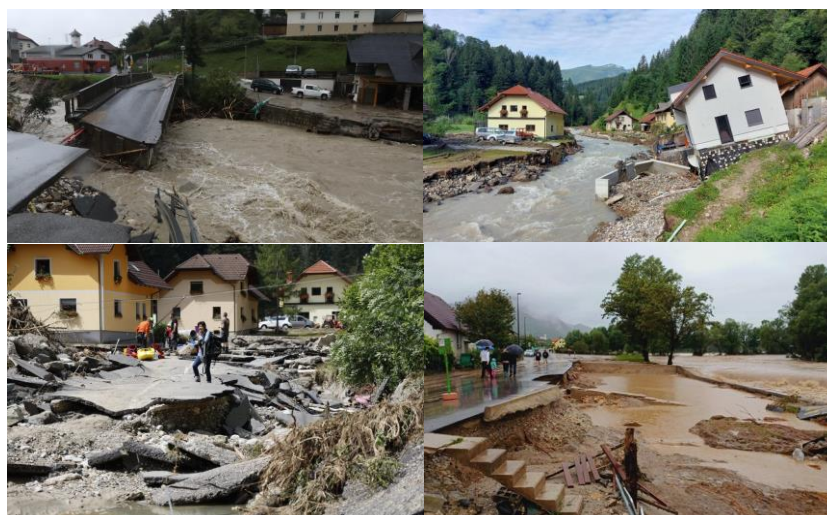
Fig. 3 The consequences of flooding on dwellings and infrastructure
