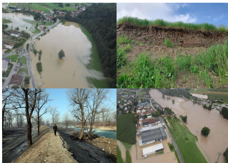
Fig. 7 The levees along the Middle Sava River section were deteriorated - there were rodent and bird tracks, as well as overgrowth that does not belong on the levees itself.
