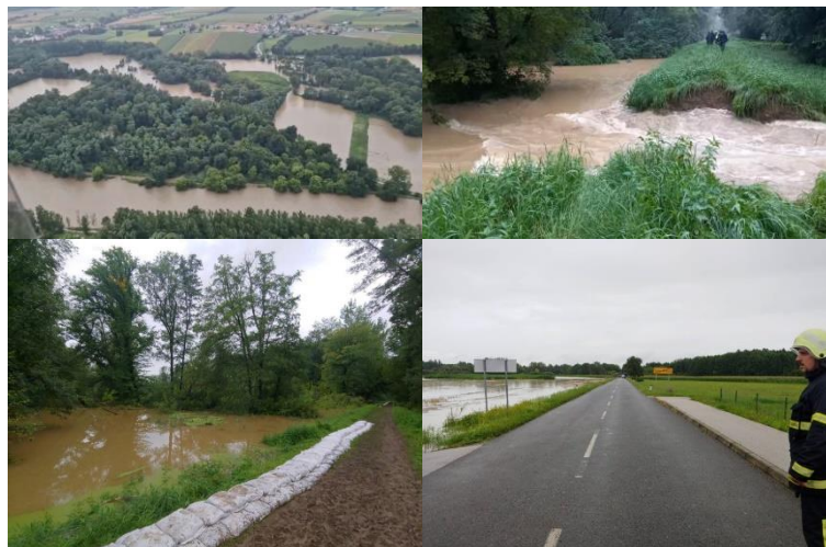
Fig. 6 Levees along the Mura needed reconstruction - but waited too long
